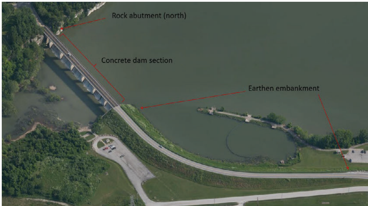
Figure 11: Lake Springfield Dam
