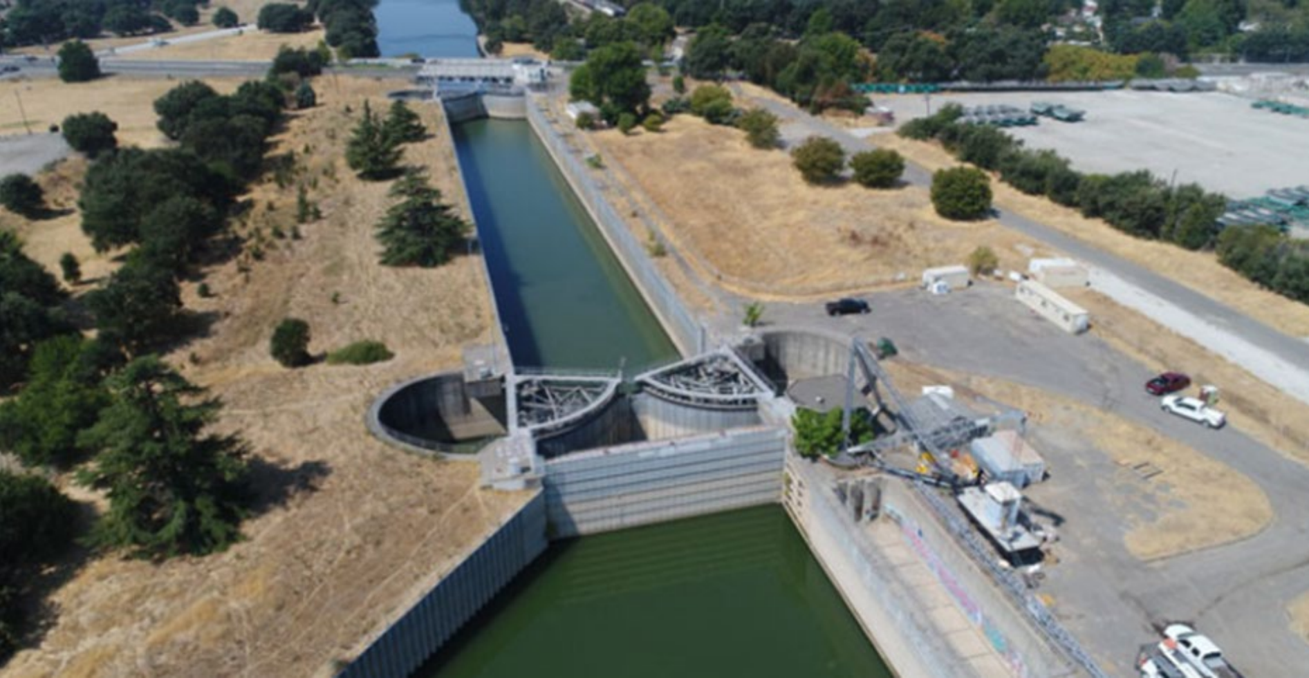
USEPA Brownfields Grant- Stone Lock Facility in West Sacramento, CA
